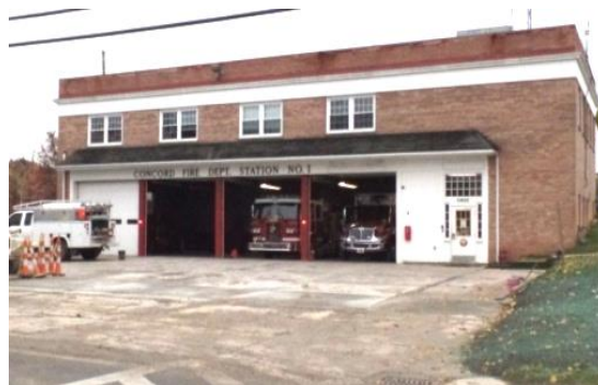
Front of Station 1
