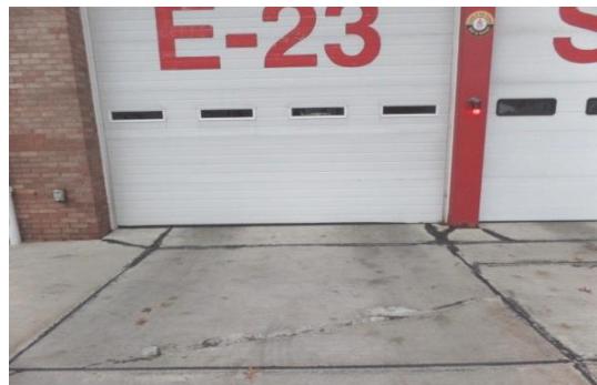
Concrete pad deterioration
