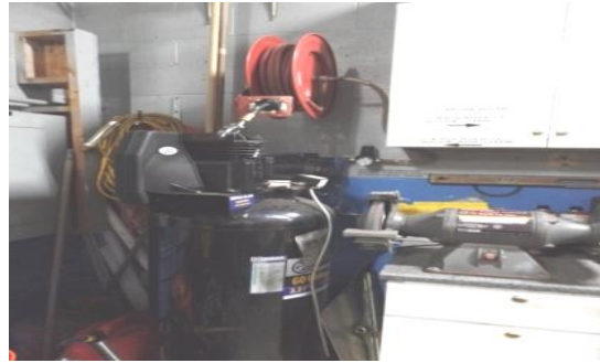
West wall; air compressor
