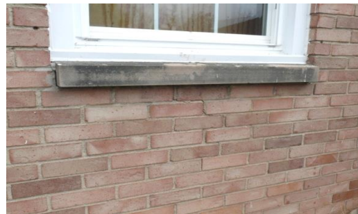
South wall mortar cracking
