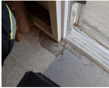
Second floor condition
