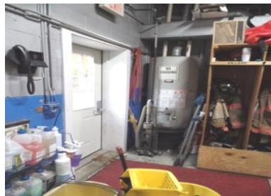
Rear of the north bay
