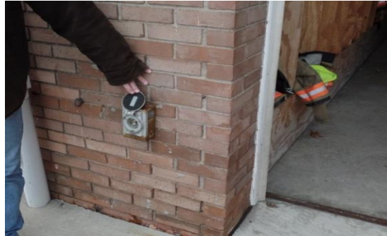
External portable generator connection
