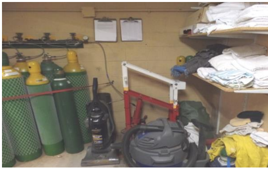
West wall storage room-oxygen cascade system
