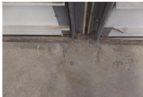
Concrete floor spalling
