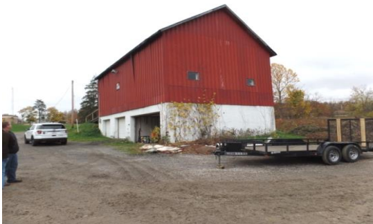
Barn storage and gator trailer
