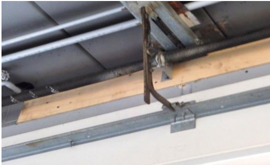
Overhead door emergency releases
