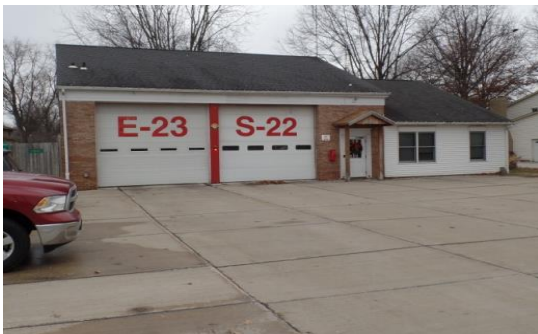
Front of Station 2
