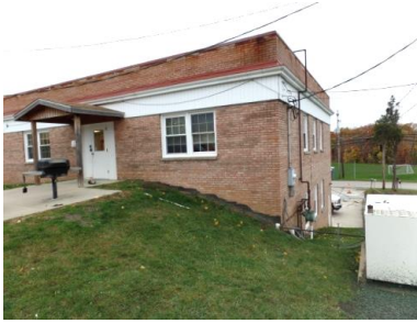
Second floor entry
