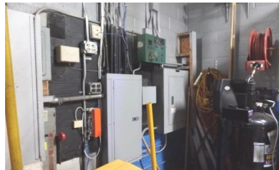
Electrical panels on south wall
