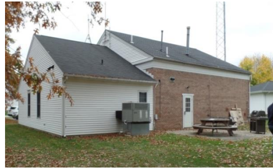
Rear of Station 2
