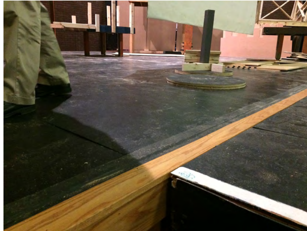
Stage floor covered with plywood due to condition
