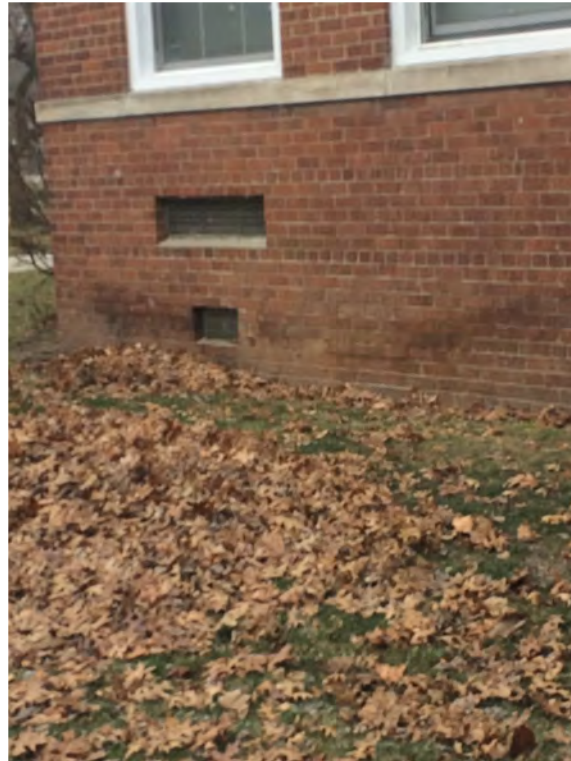
Due to new HVAC system, masonry infill needed at unit ventilator outside air grilles.
