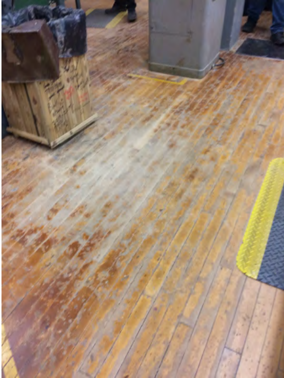
Wood floor in poor condition
